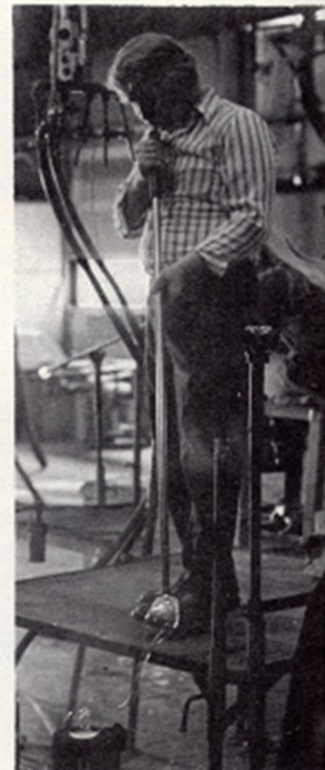
...who completes the shaping, forms the jar, and "blows the straw."
